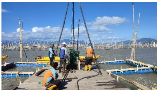
Figure 2. Machine Support Base and Drilling Machine
