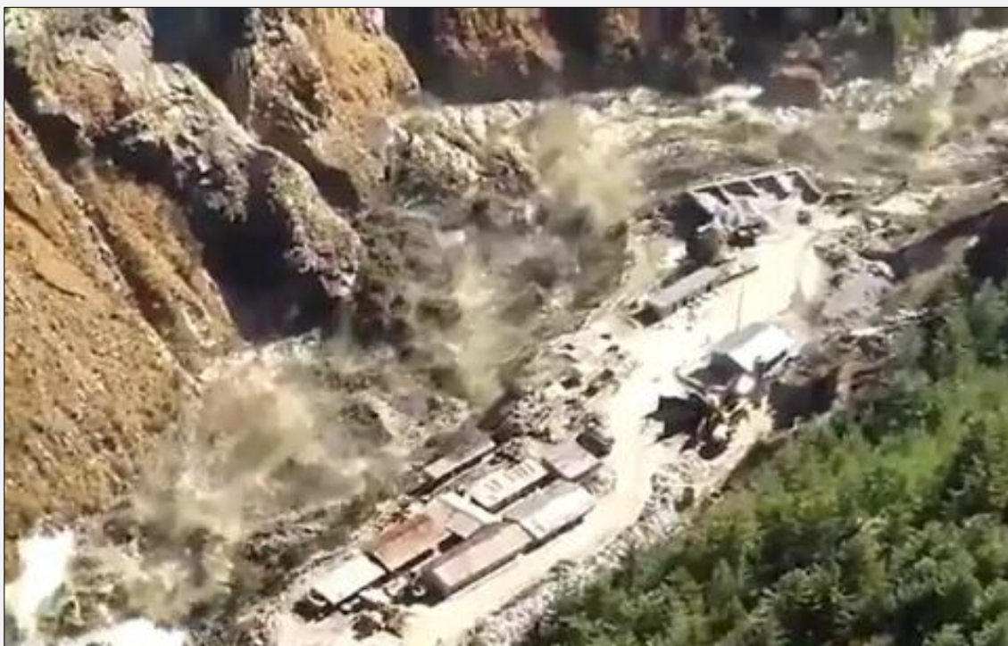
Figure 10. Image showing the debris flow along the path of Dhauliganga River, which completely destroyed the structures coming on the way
