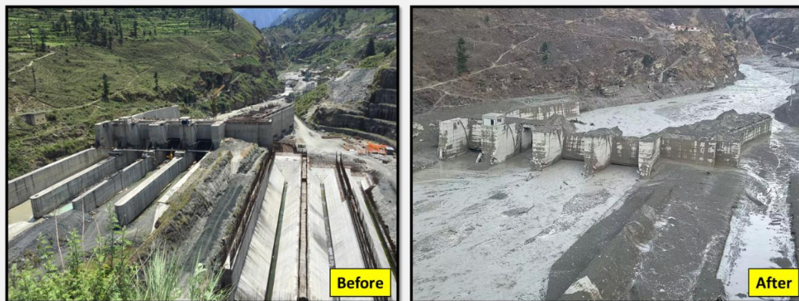
Figure 15. Before and after flash flood conditions of Tapovan Vishnugad Hydro Power Project (520 MW) clearly show severe damage to the under-construction hydropower project due to the devastating flash flood of 07 February 2021 ( Source: Before - http://webtag.ae/rithwik/view/front/modules/_portfolio/data/27/hURCWLUssu3q.JPG After - https://static.toiimg.com/thumb/msid-80738861,width-1200,height-900,resizemode-4/.jpg )
