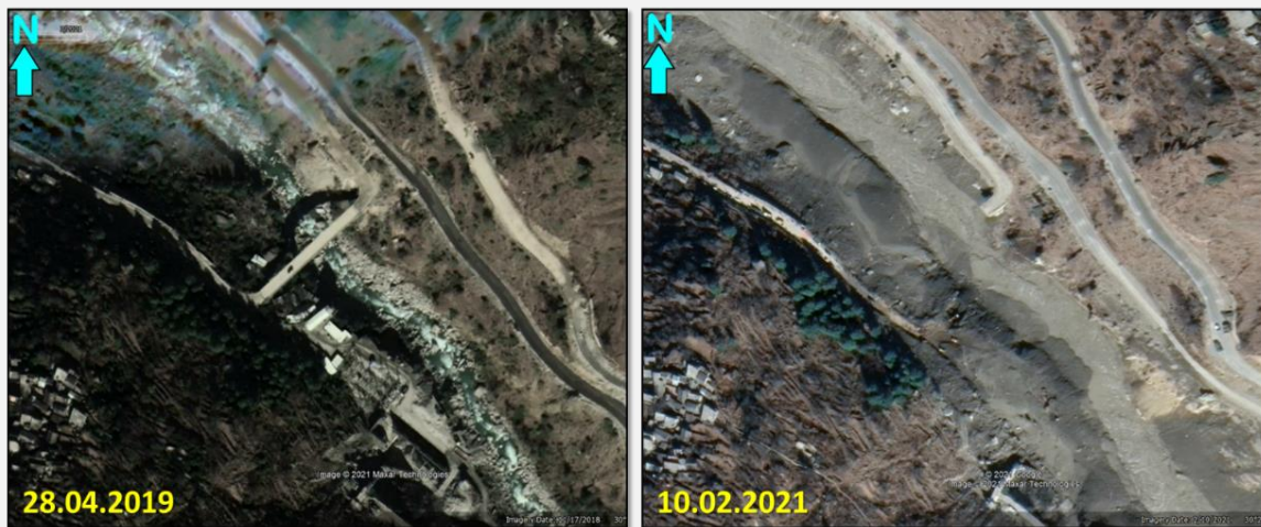
Figure 13. Pre- and post-event Google Earth images of the Rishiganga Hydro Power Project (13.2 MW) clearly show a complete washout of the operational hydropower project due to the devastating flash flood of 07 February 2021
